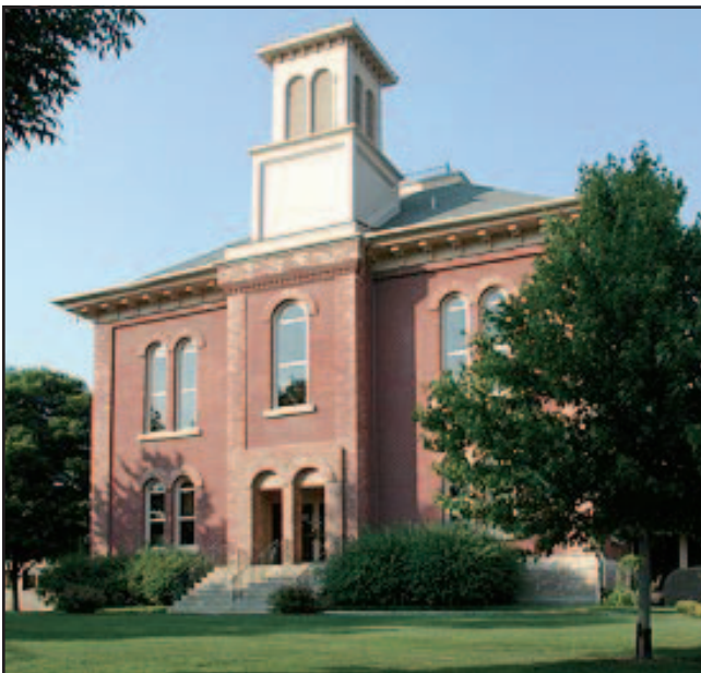
Boone County Courthouse, Belvidere
